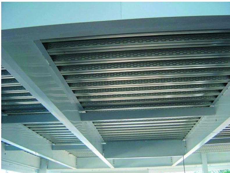
Figura 3 - Laje Steel Deck
